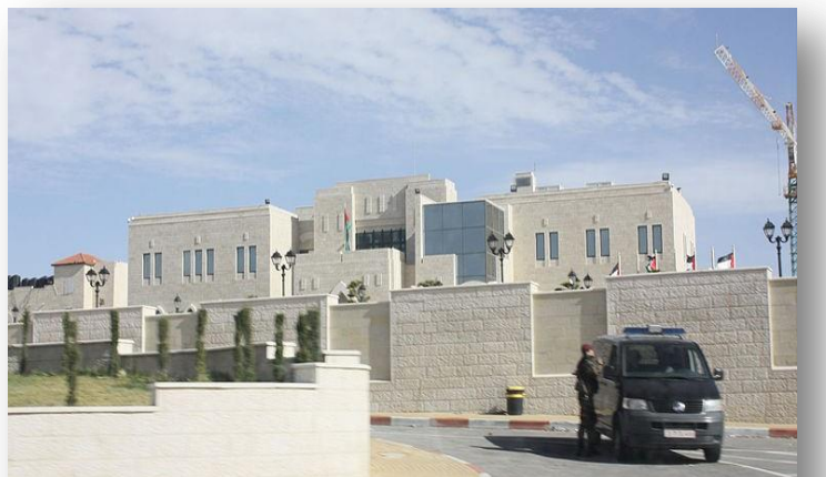
The new Presidency Premises/Ramallah
